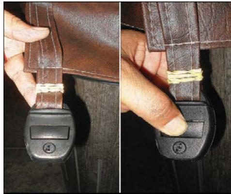
**Step 3** With the straps pulled tight (but not overly tight), lightly pre-drill the location for screw placement. Gently drill 3 holes - one for each screw slot in the lock.
